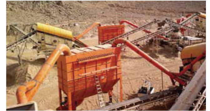
● 400TPH Crushing plant
