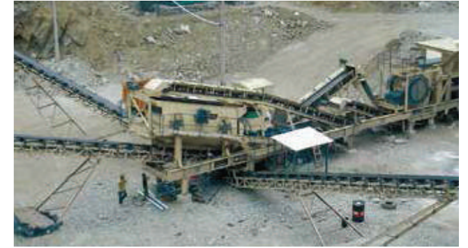
● 150TPH Crushing plant
