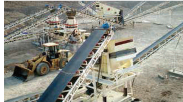
● 300TPH Crushing plant
